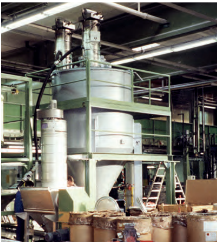
Continuous charging of a mixing container and autoclave for manufacturing adhesives.
