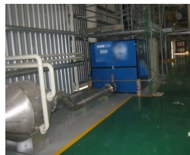
Roots blower package with air cooler set
